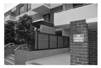
**Figure 6:** A natural ladder formed by a low-lying brick wall and parallel wooden fence leading to a walkway shade that provides easy access to the first floor balcony.
