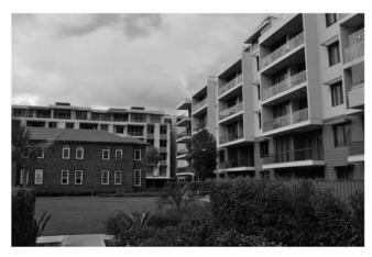
Figure 3: Glass balconies oriented towards centre of complex allow for natural surveillance of common area and landscaping.
